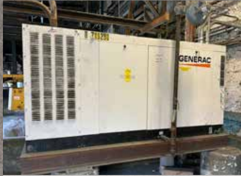
Generac 130 kW Industrial Generator, Natural Gas
